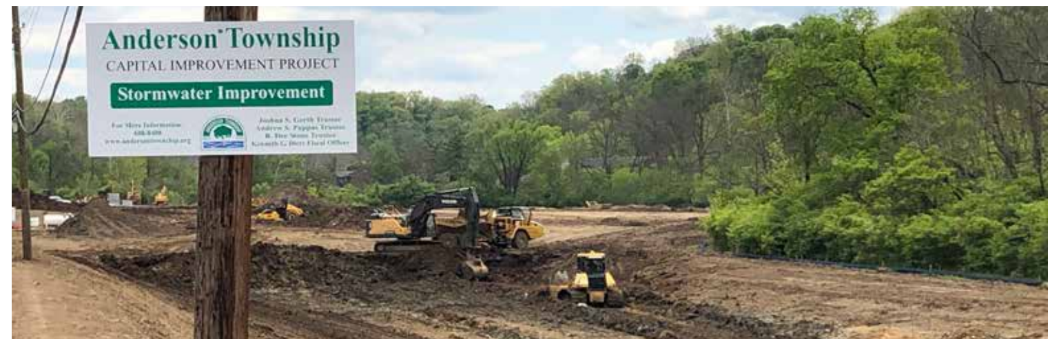
Construction has begun on the Clough Creek stormwater basin on Clough Pike, west of Newtown Road. The soil is being utilized for the adjacent Harmony Senior Living development.
