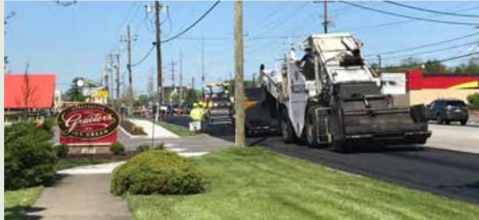
Beechmont Avenue grinding and repaving
